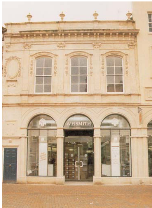
After, new shop front restores the architectural relationship between ground and upper floors
