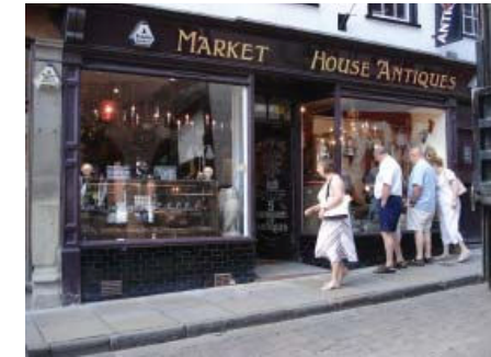
Victorian shop front in Ross with console brackets and plate glass windows
