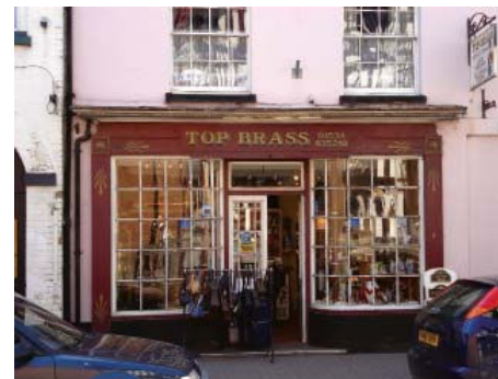
A late C18/early C19 shop front in Ledbury with deep entablature.
