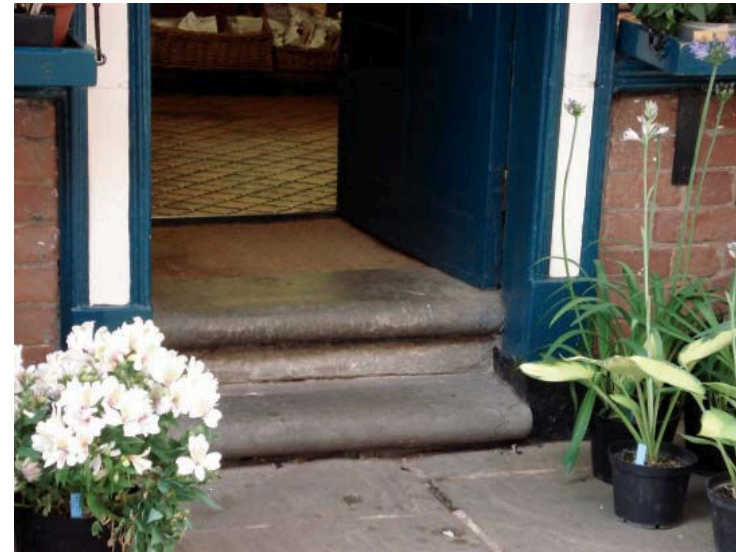
Rounded stone steps - part of the character of listed buildings. Difficult access for some customers
