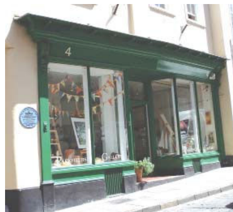
Recess doorway and deep glazing bars project light and shadow over shop front
